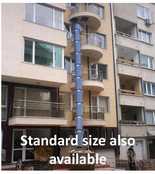
MR HIRE RUBBISH CHUTES ARE MANUFACTURED OF HIGH DENSITY POLYPROPYLENE 750MM ID TUBE SECTIONS SPIGOTED, CHAINED AND BOLTED TOGETHER. THE MAXIMUM RECOMMENDED LENGTH IS 30 METRES AND THE CHUTES CANNOT BE BENT OR TWISTED IN ANY MANNER RATHER MUST HANG VERTICALLY. DUE TO THE PARTICULARITIES OF EACH CHUTE ALLOW 10 WORKING DAYS FOR DELIVERY.
